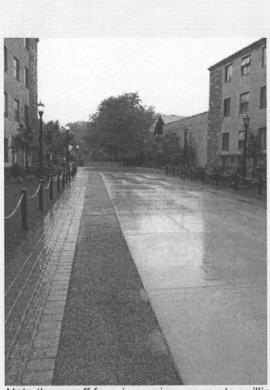
Note the runoff from impervious concrete spilling over to the pervious concrete
